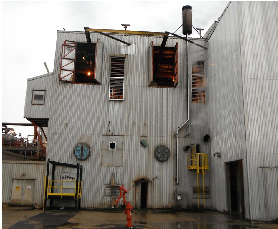
**Figure 5: Upper hoist access doors on Ammonium Plt. #1 Compressor Bldg.**
